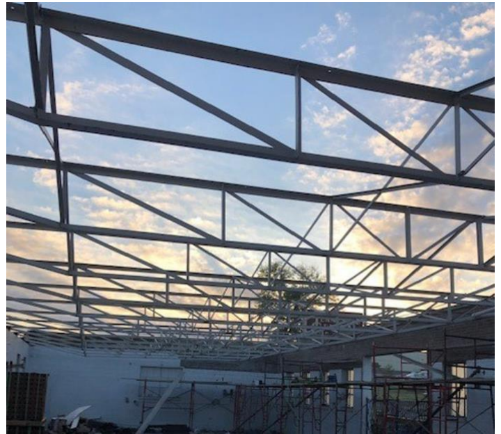
New Trusses Installed photo submitted by Terry Bebout
