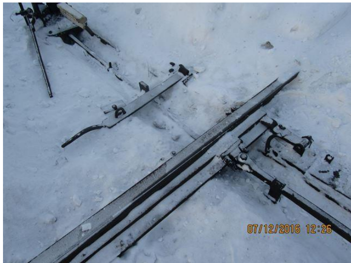
The switch with the problem
