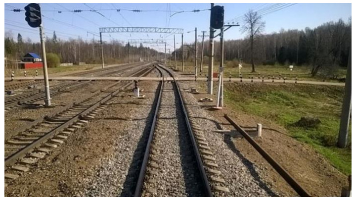
Uski station, station building, platform, tracks
