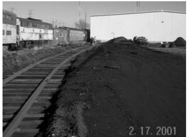
TCRM has gotten approval from Tennessee Commercial Warehouses to extend 1 of our tracks farther eastward to the west wall of their warehouse. TCRM's track Supergang has dug roadbed, placed ties, bolted rail, installed a bumping post, spiked some of the rail already. A few more Monday/Saturday work sessions & we're ready to spread ballast & level track!! In this digital photo by **Terry Bebout** the gang is installing the bumping post and preparing to spike rail.
