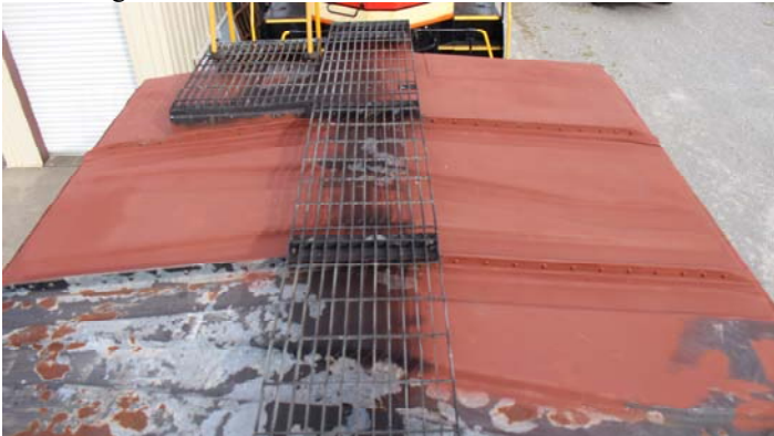
View of TCRX 1155 roof area described above
